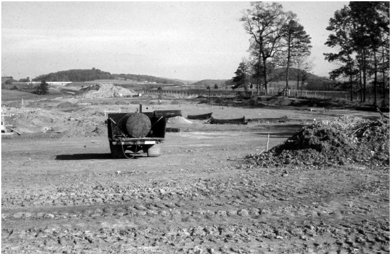
original excavation of campus
